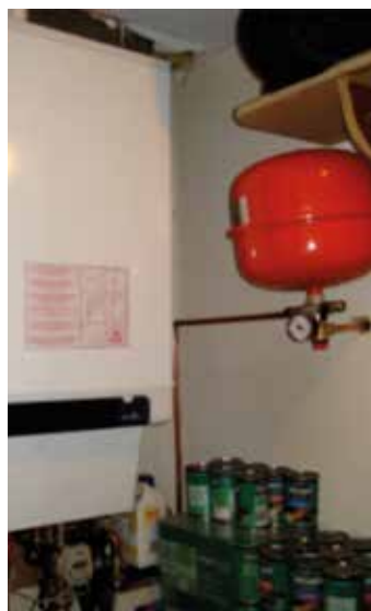
Figure 33: Picture of the indoor hybrid gas boiler and heat pump module (field test setup).
