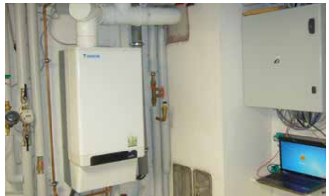
Figure 38: Picture of the installed indoor unit of the hybrid.
